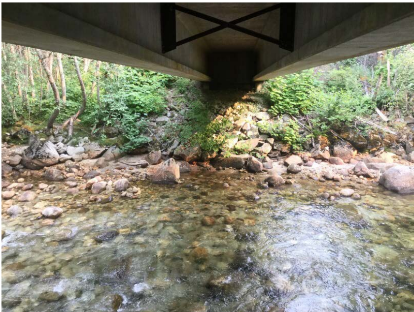
Left Bank Abutment when facing downstream
