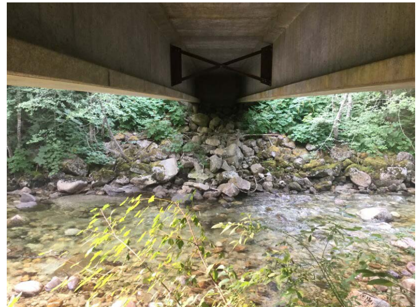
Right Bank Abutment when facing downstream
